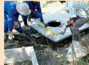
Construction of a C-section precast VIP
