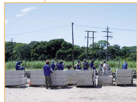
Figure 6.8 Ugu community workers in the precast yard
