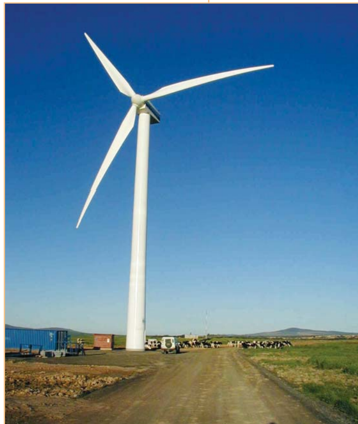
Figure 6.19 Klipheuwel wind farm
