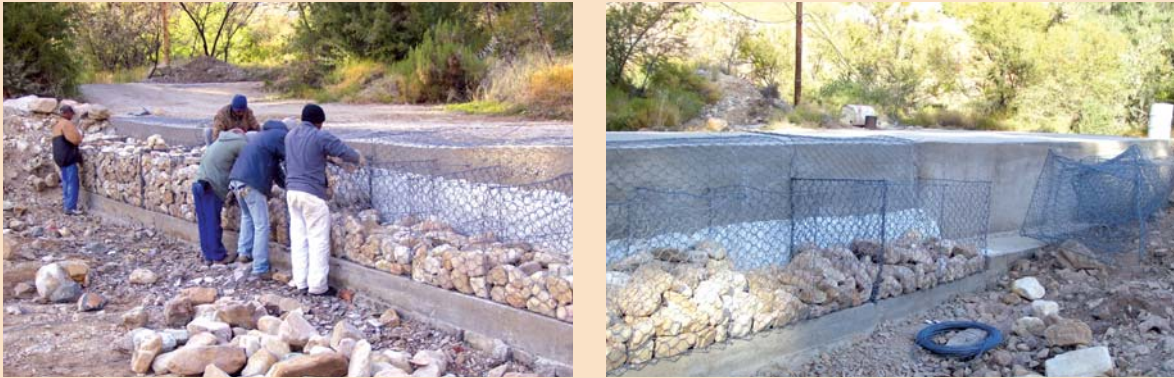
Gabions being put in place to protect the bridge
