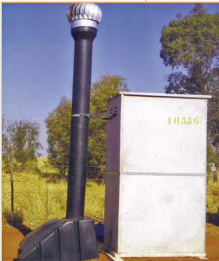
Figure 6.6 The biological latrine with black unit facing north
