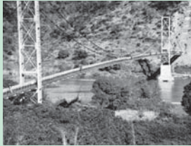
Pipeline suspension bridge over the Umgeni river (1961)
