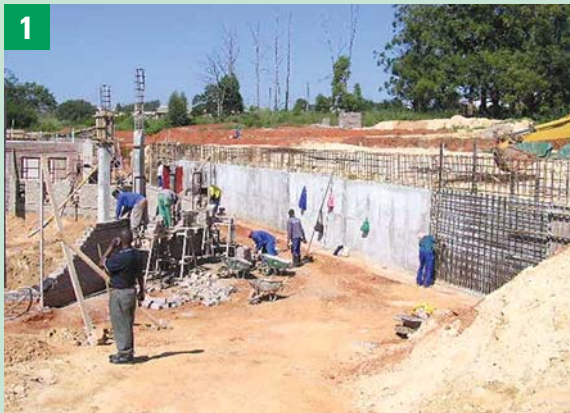
Slow progress in early 2006
