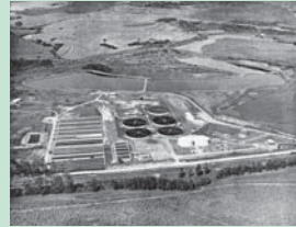
KwaMashu sewage disposal works (1965)
