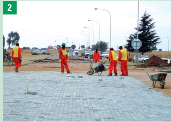
New paving being laid
