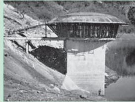
New intake tower for the third aqueduct – Nagle dam (1964)
