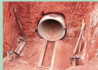
Pipe jacking across the R40
