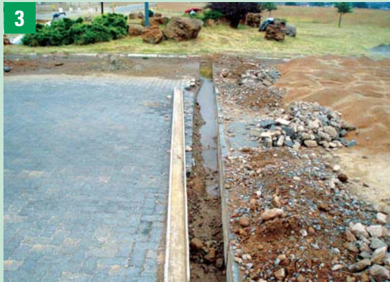
Joint under repair
