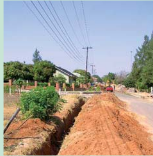
Broken pipes being replaced
