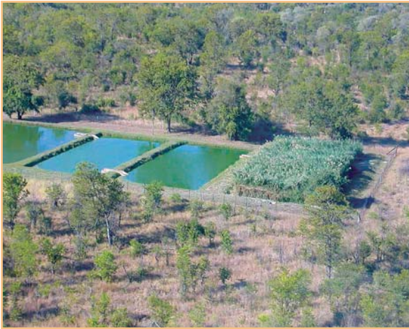
Figure 6.10 Reed-bed for nutrient removal and final polishing – Punda Maria rest camp, Kruger National Park
