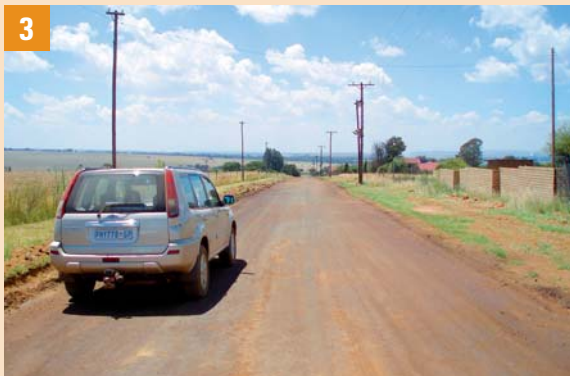
The completed road
