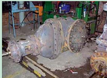
Removed and repaired
