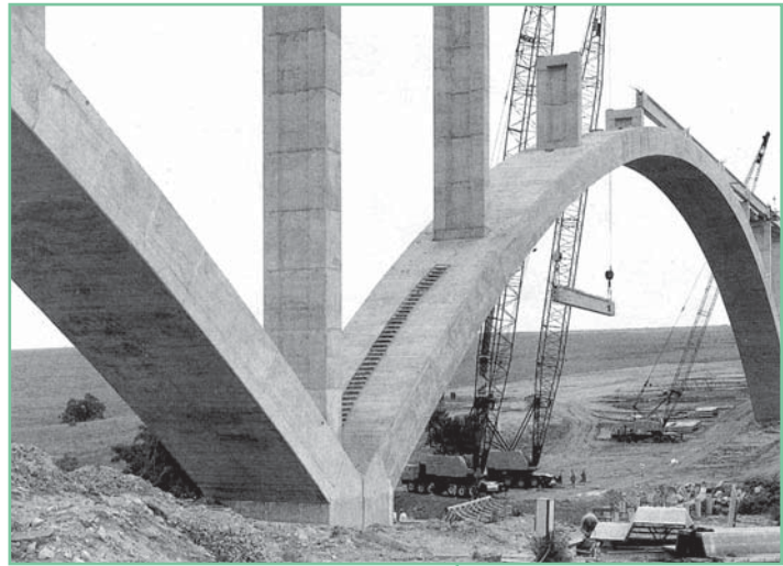
Figure 2.13 Construction of arch bridges to support the new Diepsloot sewer – a massive development in the 1970s to accommodate long-term residential expansion in the northern suburbs
