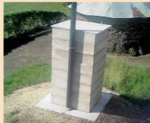
Completed new C-section precast VIP
