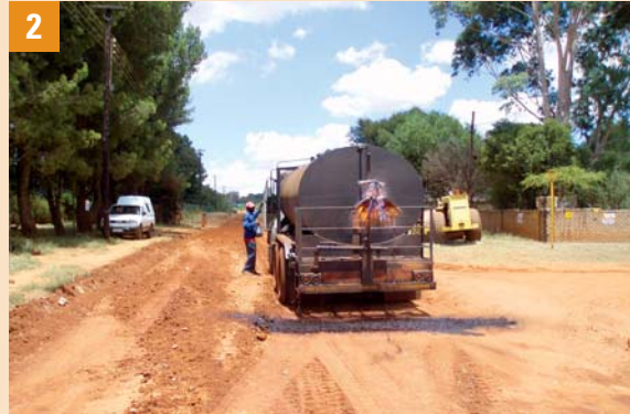
Stabiliser being applied
