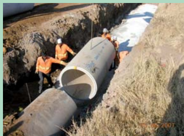
Laying stormwater pipes
