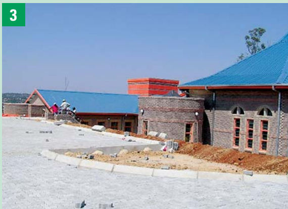
Civic centre nearing completion
