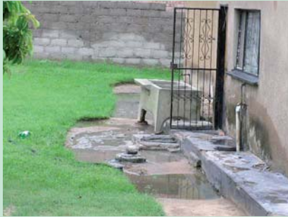
Sewage bubbling out in the back garden
